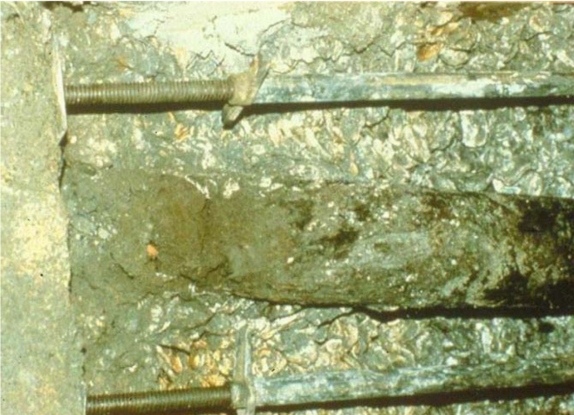
Figure 1. Examples of Wood Piles That Have Suffered Substantial Rotting
