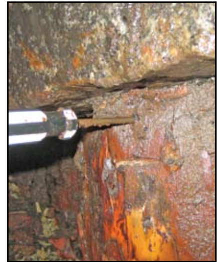
Figure 3: Piles should be probed from various angles and penetration depths should be recorded.
