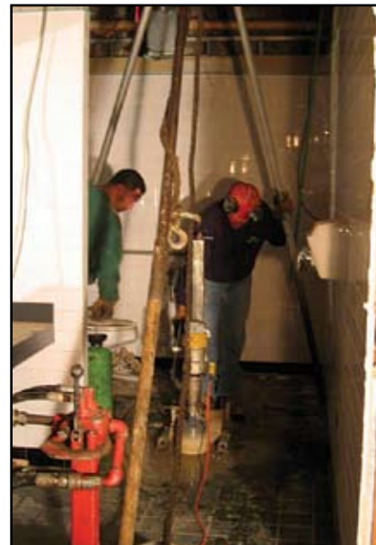
Figure 2: Installation of an observation well on the building interior.
