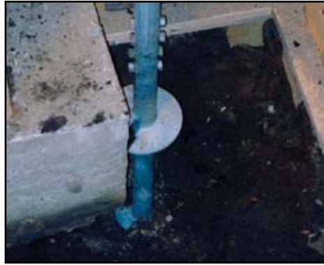
Figure 7: Helical pile is installed adjacent to the existing footing.
