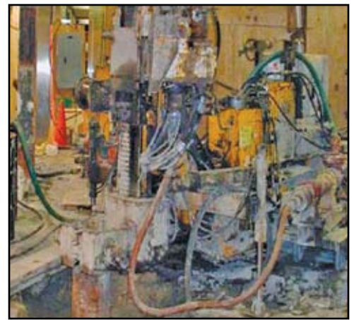
Figure 5: Mini-pile installation can be messy and disruptive.
