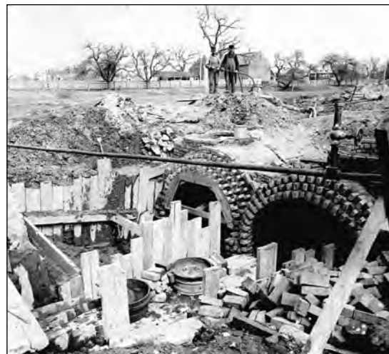
Courtesy of the Boston Water and Sewer Commission
