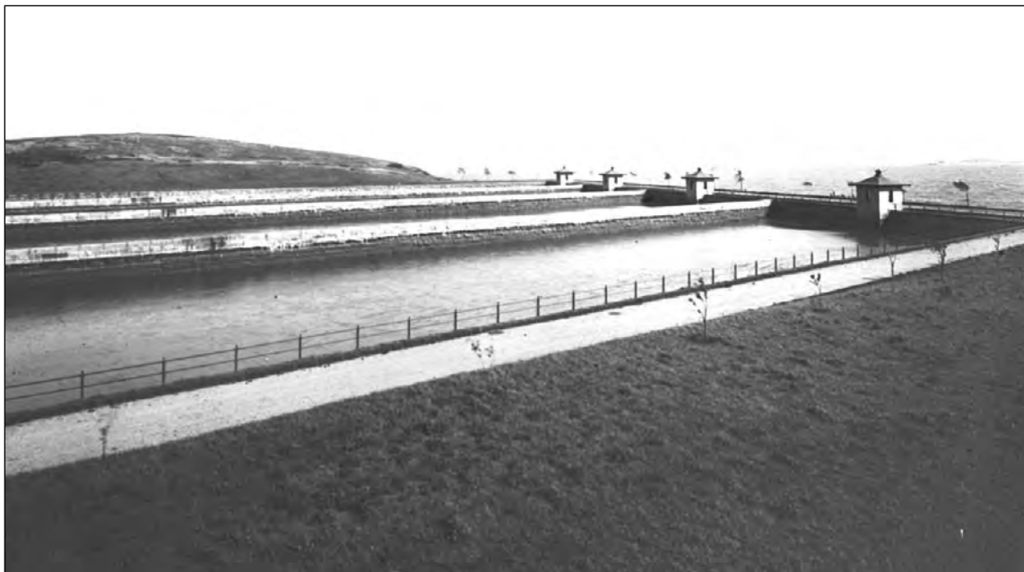
Moon Island sewage reservoirs showing houses for flushing gates, about 1900.
